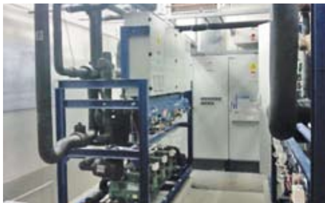
Kaufland CO 2 /HFC-134a cascade system installed in Croatian shopping center in Vukovar
