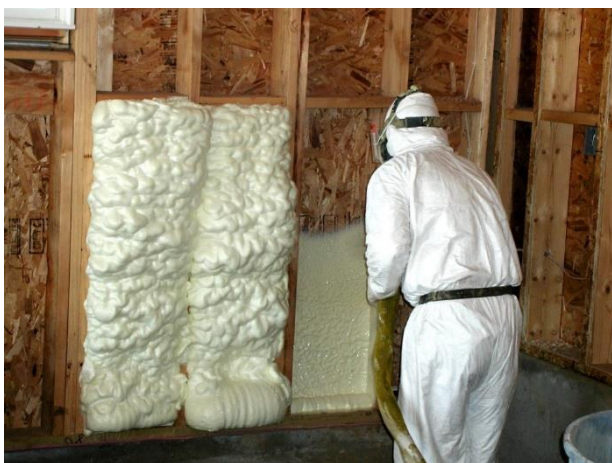
Spray foam installation
